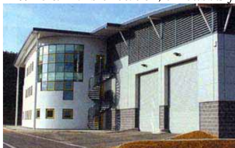
Materials Recovery Facility, Norfolk
