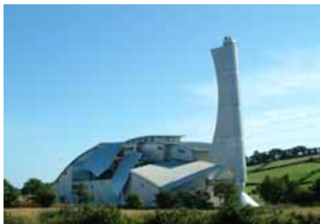
Energy from Waste, Isle of Man
